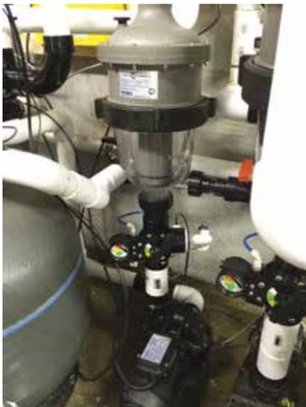
*Waterco's multi award winning, MultiCyclone technology is incorporated into the Hydroxypure system. It maximises the strength of sanitisation by cleverly performing the dual role of mixing the ozone into the pool water and then providing adequate contact time with the water to be fully effective.*
