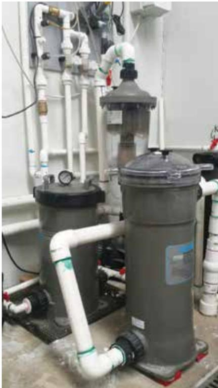
Waterco's MultiCyclone centrifugal filter and Trimline Leaf Trapper.
