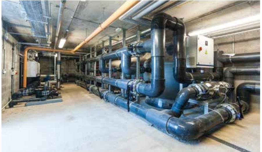
▲ Five SMD1800 Micron commercial sand filters were installed for the main pool and one SMD1800 Micron commercial sand filter was installed for the children’s splash pool.
