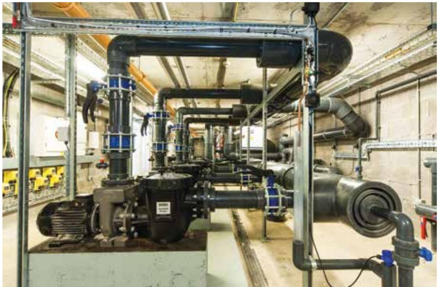
▲ Four 7Hp BH5000 Cast Iron Pumps were installed for the main pool and two Hydrostar 6HP pumps for the children’s splash pool.
