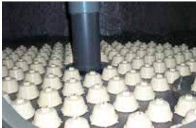
Nozzle Plate underdrain system
