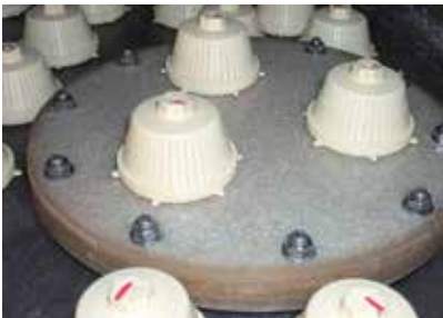
Internal Nozzle Plate Service Hatch
