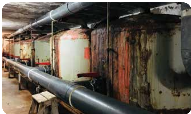
Corroded metal fabricated filters
