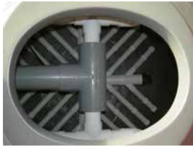
Lateral underdrain system
