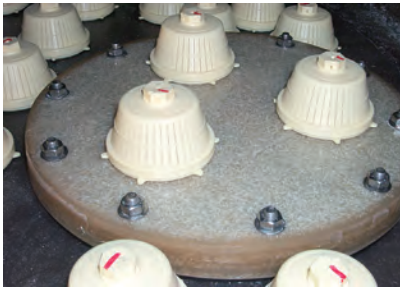
Internal Nozzle Plate Service Hatch
