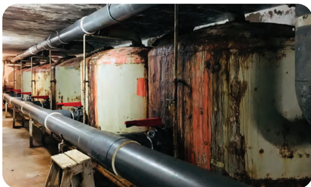
Corroded metal fabricated filters
