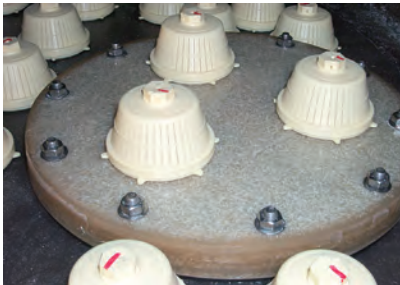
Internal Nozzle Plate Service Hatch
