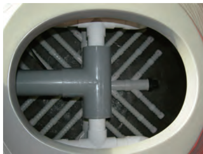
Lateral underdrain system
