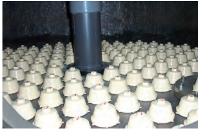
Nozzle Plate underdrain system
