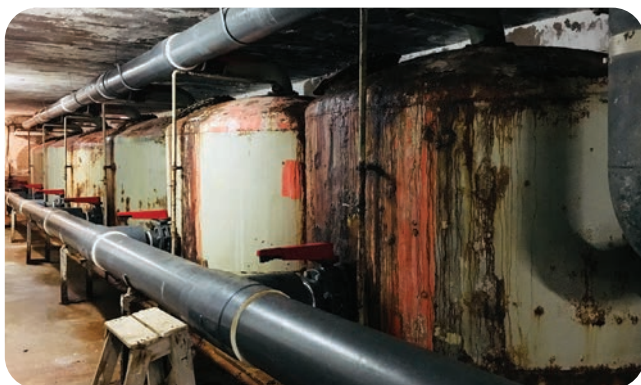
Corroded metal fabricated filters
