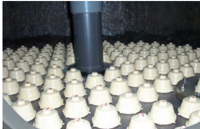
Nozzle Plate underdrain system
