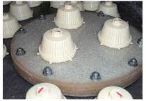
Internal Nozzle Plate Service Hatch
