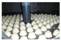
Nozzle Plate underdrain system
