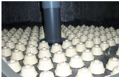
Nozzle Plate underdrain system
