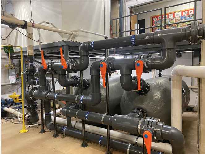
Waterco's new lateral configuration provides a more natural flow of water through the filter, ensuring optimum water filtration and balanced fluidization of the filter bed during backwashing.
