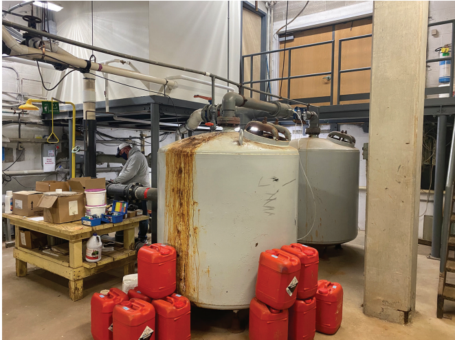
An ageing filtration system was affecting pool water quality and the health of swim school students who trained regularly at the facility.
