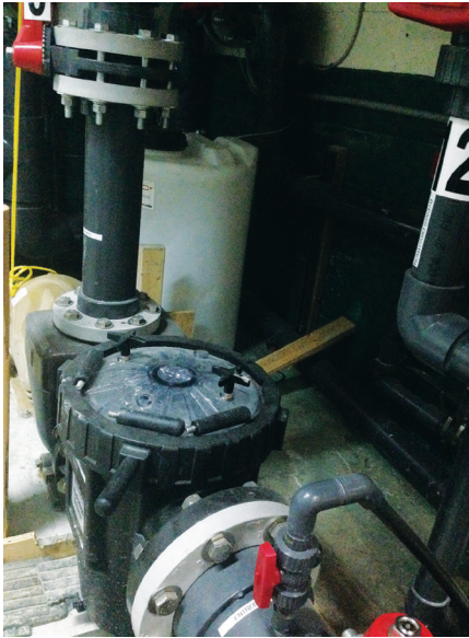
Hydro 5000 pump features a hydraulically efficient bronze impeller which allows for quiet operation and excellent flow plus an 18 litre thermoplastic strainer.
