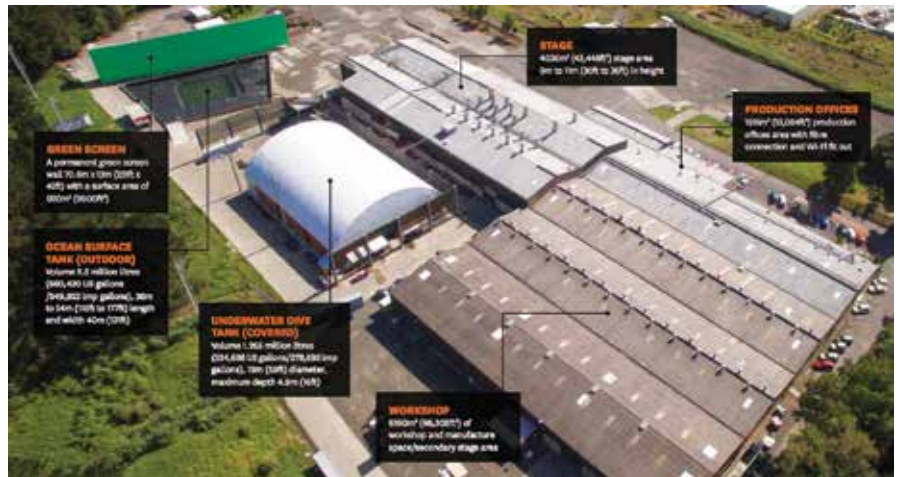
Kumeu Film Studios, 27 hectare site with and 1.267 million litre indoor and 2.5 million litre outdoor dive tank.
