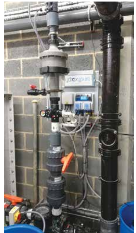
Hydroxypure sanitisation is based on the Advance Oxidation Process. (AOP), which combines Perox, a chlorine free sanitiser ( H_2O_2 ) and hybrid ozone ( O_3 ) to create one of the most powerful oxidisers in nature.
