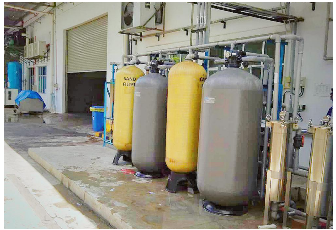
Site inspection & on-site training
